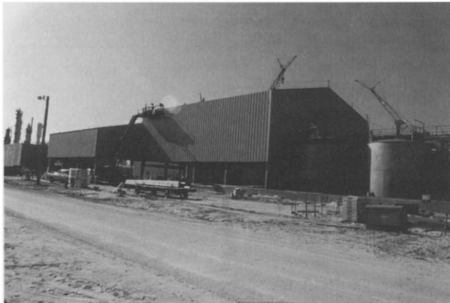
Fig. 7. Construction state of tank farm and waste receiving areas (February 1989).
